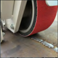
Weld seam and heavy sheets grinding
